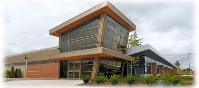
Technology Centre expansion
